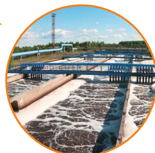
Sewage treatment plant
